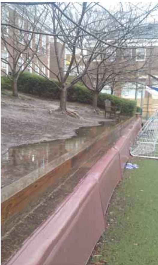
excessive stormwater runoff and erosion
