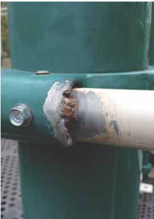
rust damage and potential hazards
