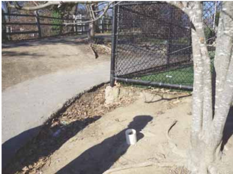
scouring from runoff
