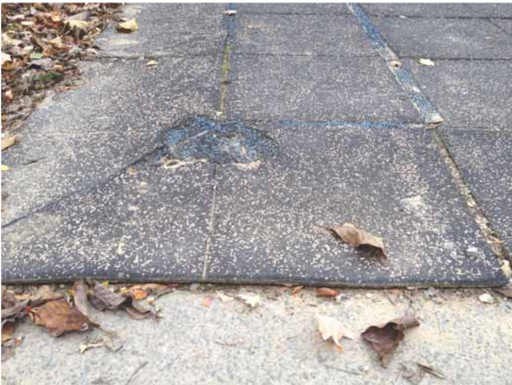
warping and peeling safety surface
