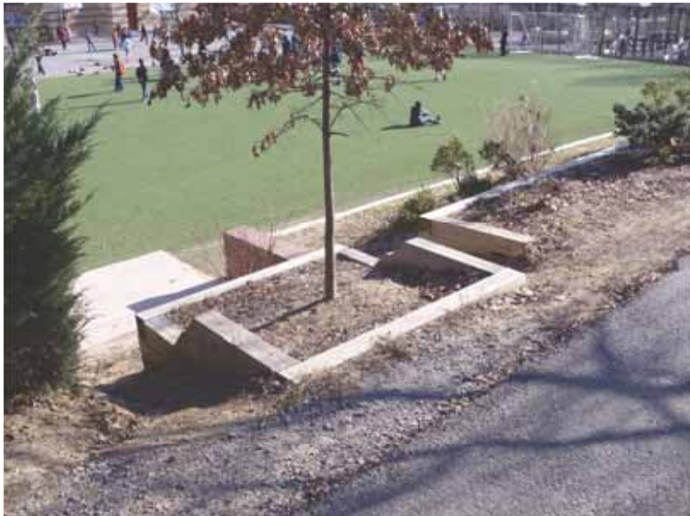
scouring from runoff and foot traffic
