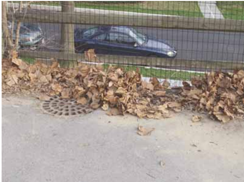
storm drain by eastern slope
