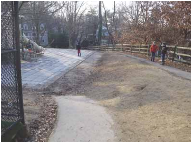
collection point for large amounts of runoff
