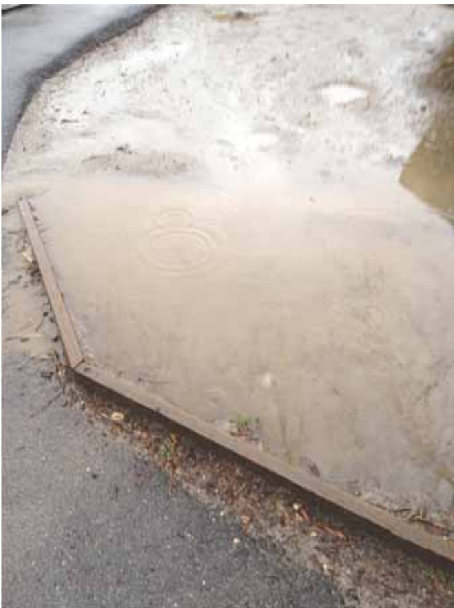
excessive stormwater runoff and erosion
